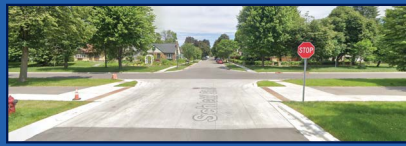
Along Wheelock Pkwy, Tabled Crossings Are Frequently Used along the Grand Round
