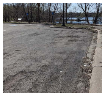
Improve parking lot pavement
