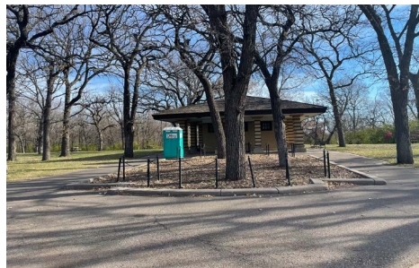
Facing east; restroom building
